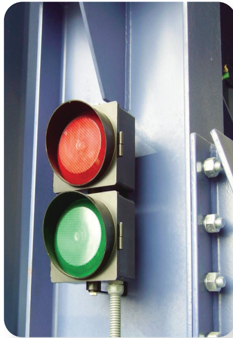
Semáforo Traffic light
